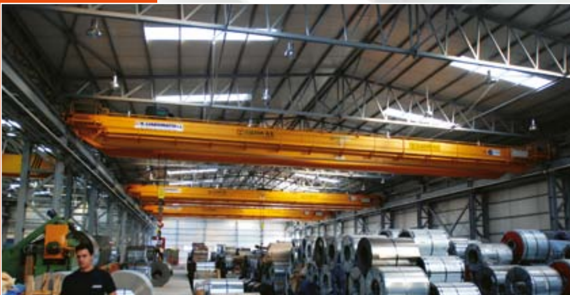
Double girder cranes 32-25-20t x 29m (Sidma S.A.)
