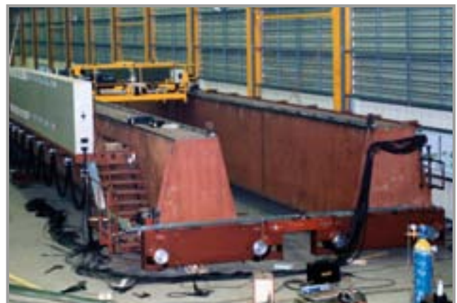
Construction of crane box
