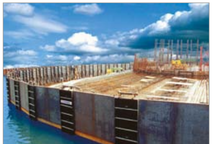
Steel retaining wall (Gefyra Joint Venture)
