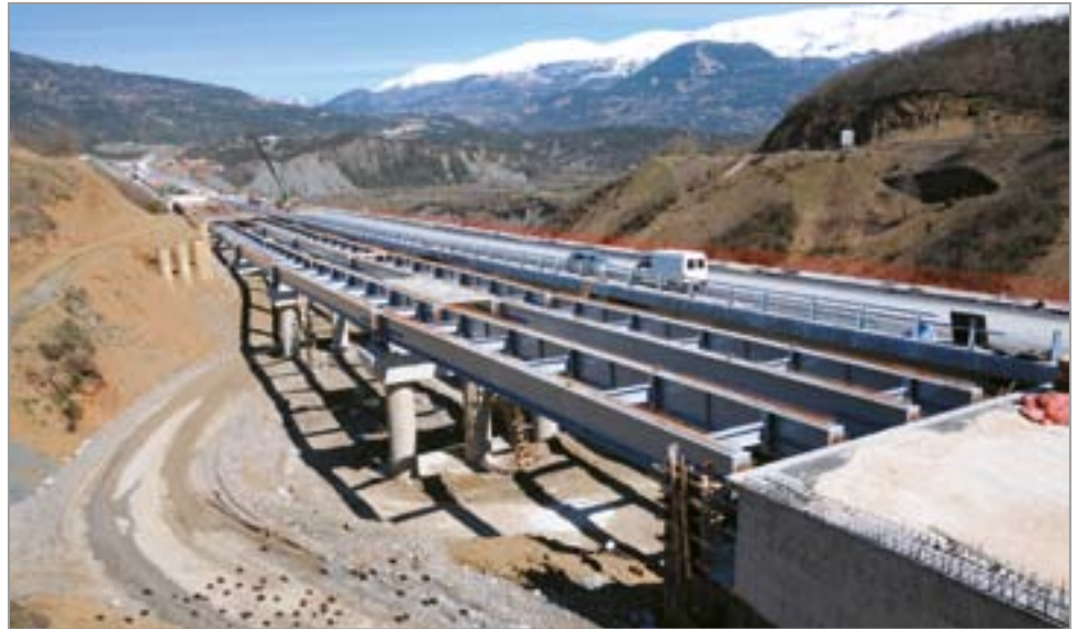
Bridge T8, Egnatia Highway Road (AEGEK S.A.)
