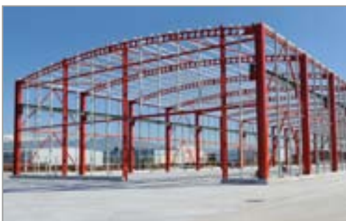
Curved castellated roof
