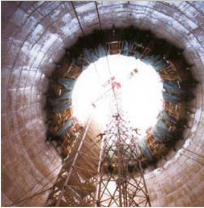
Staircase (Gefyra Joint venture)
