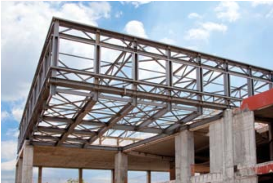
Complex of Offices (NotosCom)
