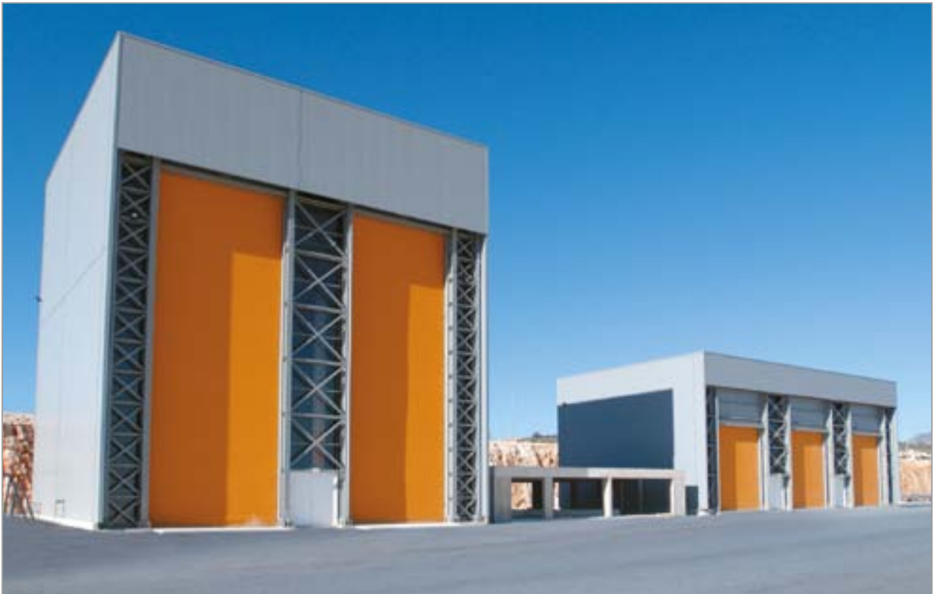
Carriers workshop (Astakos Terminal Joint Venture)
