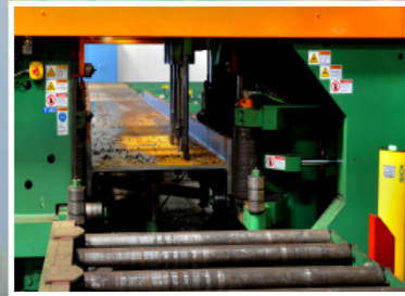
Beam Drilling Line
