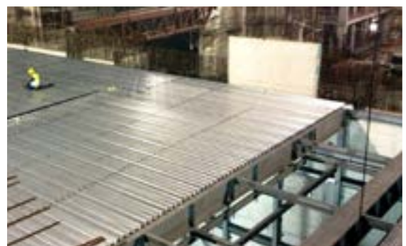
■ Built-Up Welded Beams with a total length of 11m
