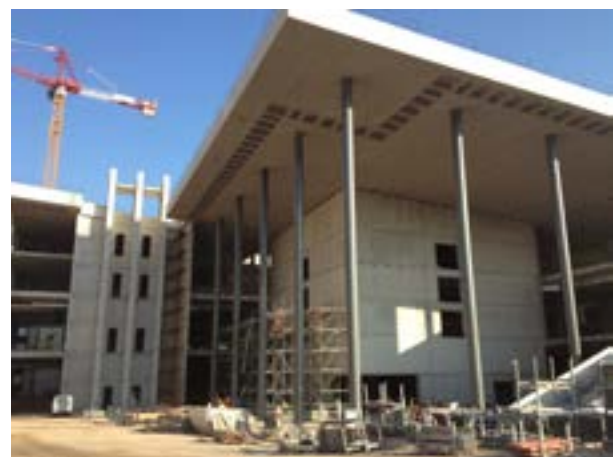
■ Built-Up Welded Beams with a total length of 27m
